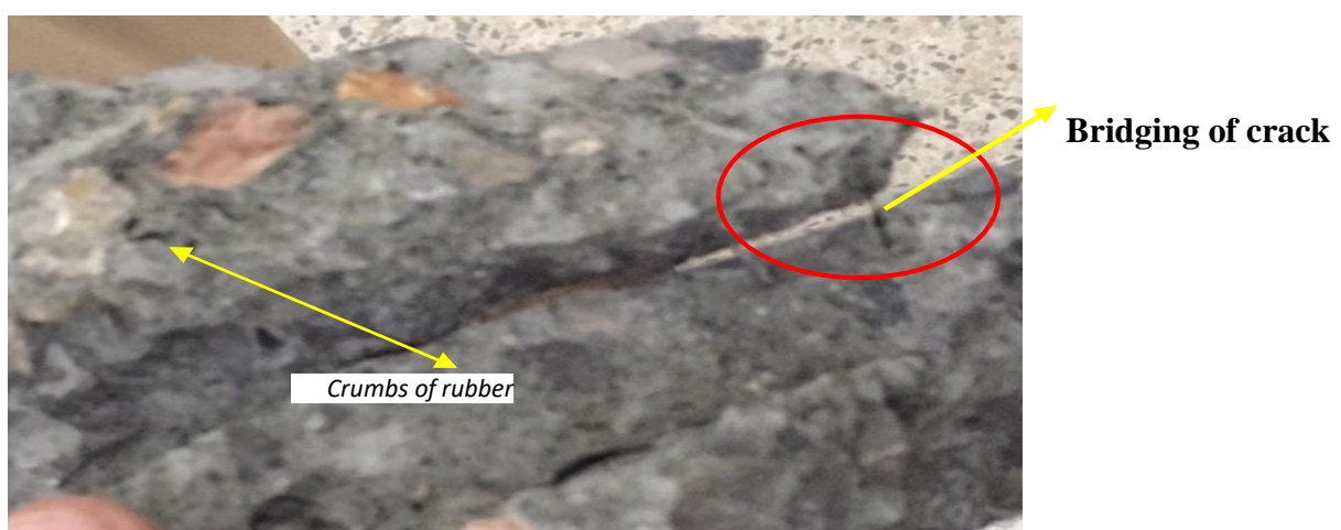
Fig. 6 Chunks of concrete bridged via crumb rubber
